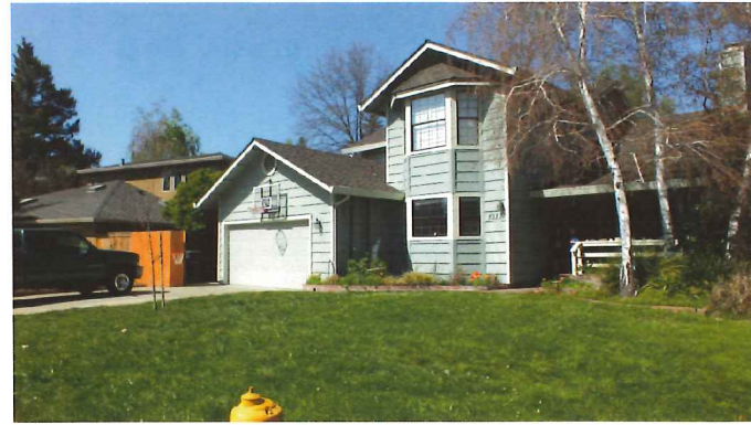
5117 Sandburg Drive - Close View from Southeast
