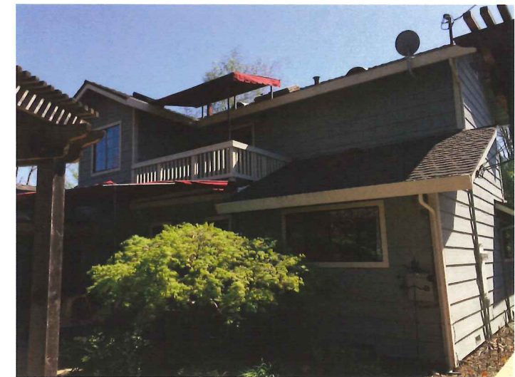
Rear yard - Closer View from the Northwest
