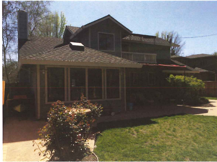
Rear yard - View from the Northeast
