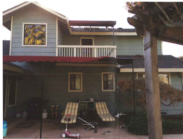
Rear yard - View from the North
