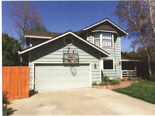
5117 Sandburg Drive - Close View from Southwest
