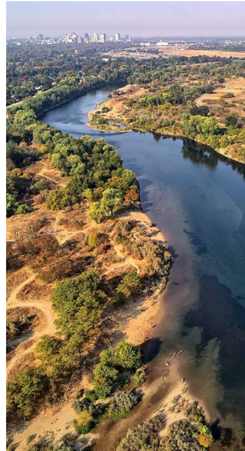
Aerial view of the Paradise Beach and Cal Expo Areas. Photo Credit: John Hannon
